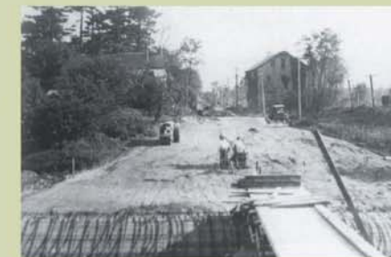
c. 1930 view looking north toward Lickdale to the widening and paving of what would become SR 72. The structure on the right is the 3-story stone grist mill at Lickdale. Photo courtesy of Francis Ditzler in "From Lickdale into the Swatara Gap," produced by the Lebanon County Historical Society.
