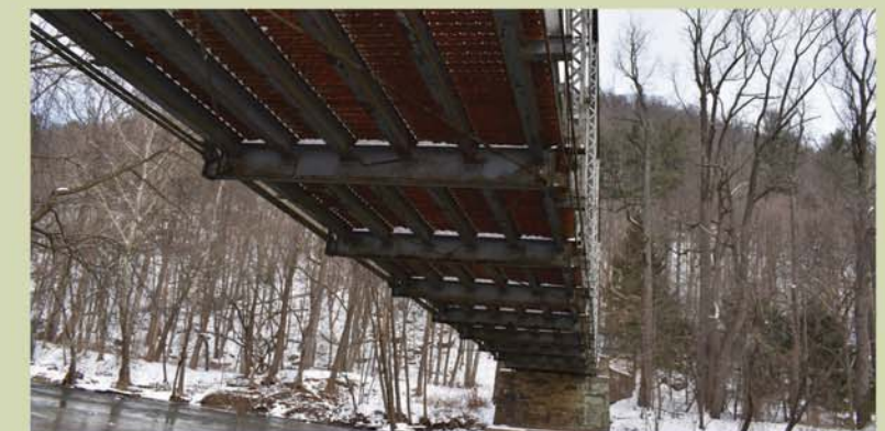
View beneath Inwood Iron Bridge at former location showing the floor beams and support system. Every other floor beam (those with lattice built-up verticals) have the distinctive Z-hanger detail.
